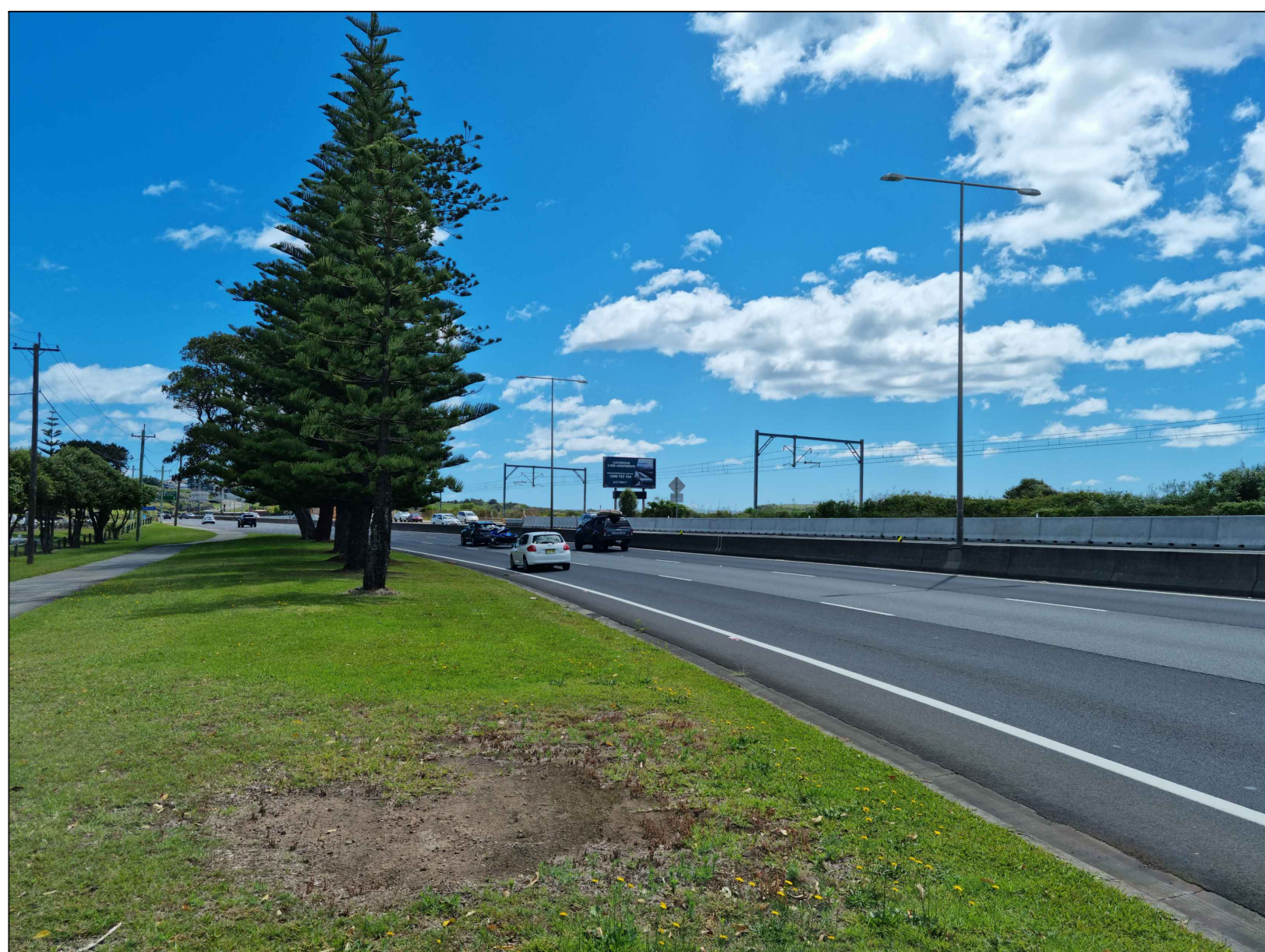
VIEW TOWARDS N-E
